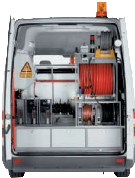
Test van with three phase HV cable
